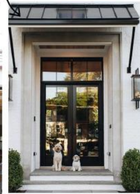
BLACK STANDING SEAM METAL ROOF WITH BRACKETS
